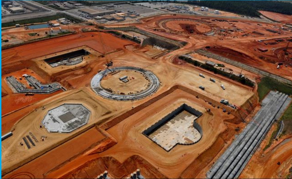
Aerial photograph of Vogtle 3 and 4 construction site. Unit 3 is located at left and top of photo and Unit 4 to the right and bottom. Heavy lift derrick crane foundation in center. August 11, 2011
